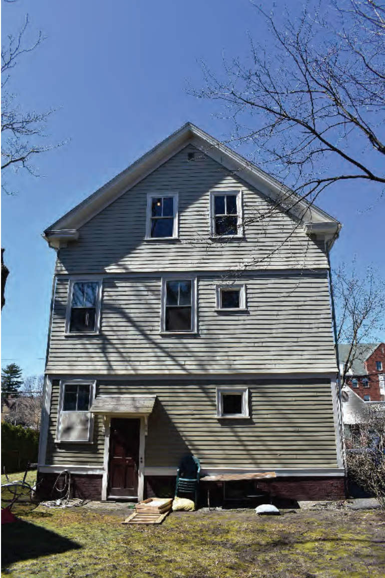
East elevation, looking west.
