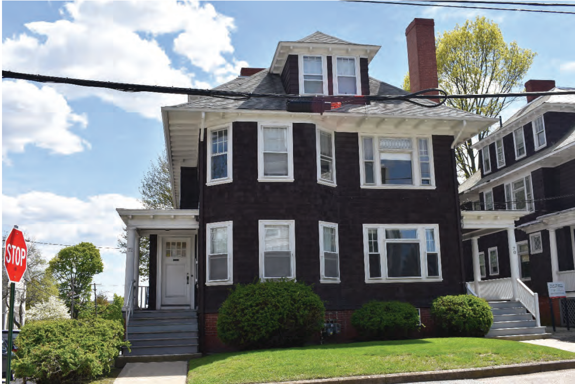
North elevation, 70-72 Charlesfield Street, looking south.
