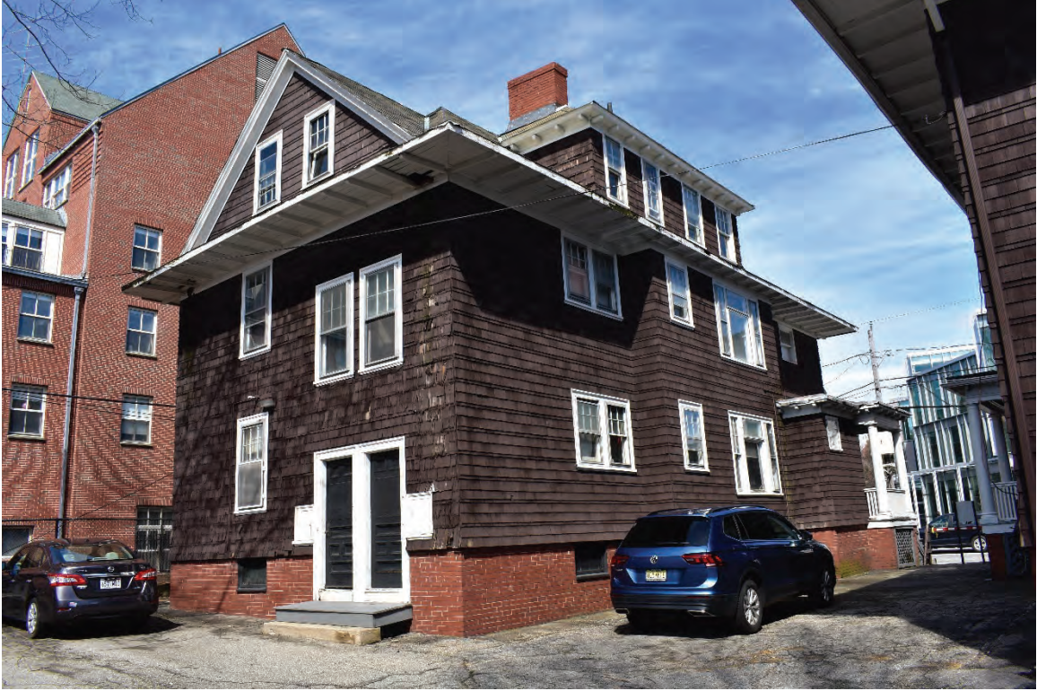
South and east elevations, looking northwest.
