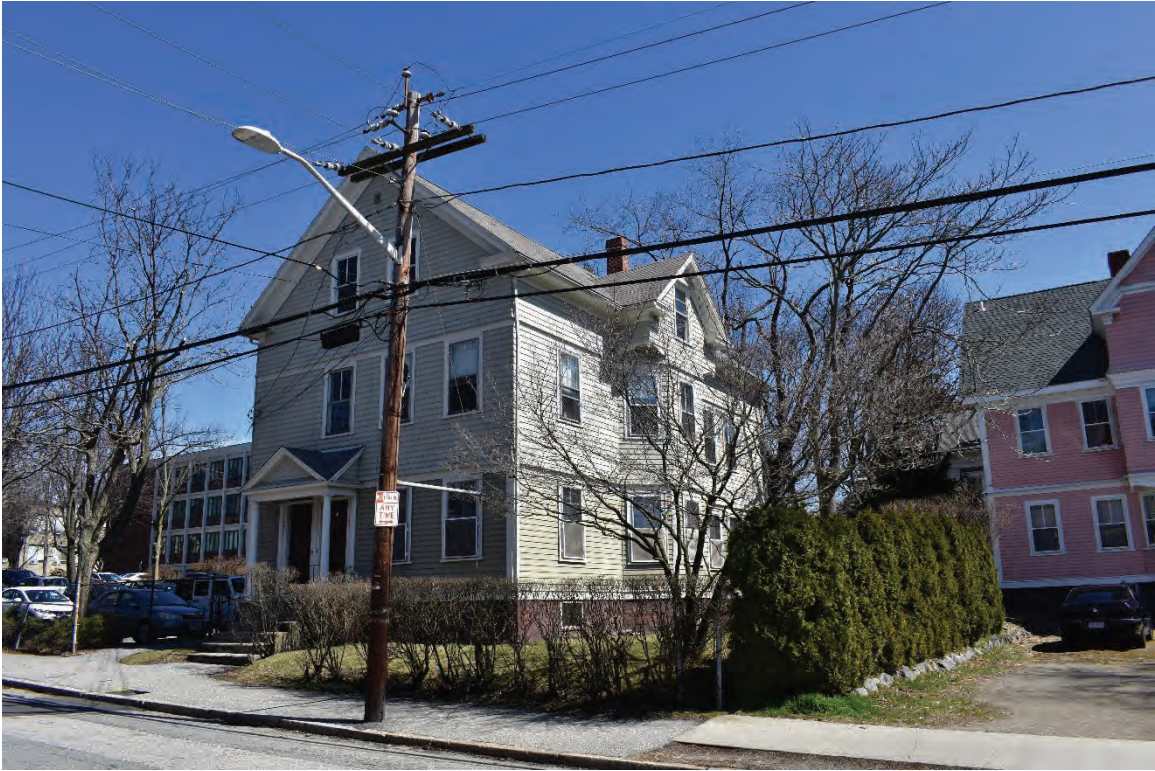
245–247 Brook Street, west and south elevations, looking northeast.
