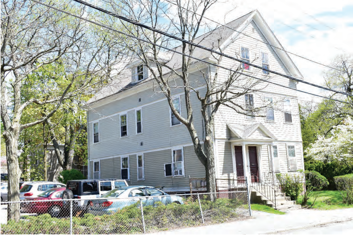
245–247 Brook Street, west and north elevations, looking southeast.
