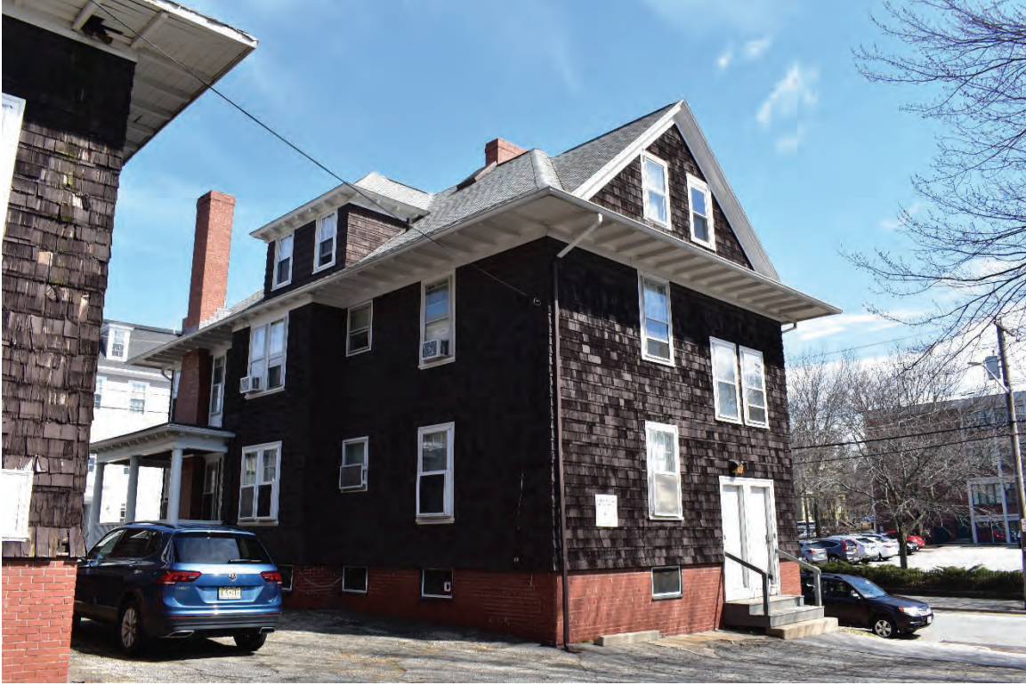
South and west elevations, looking northeast.
