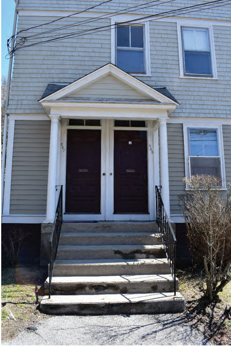
Detail of front doors, looking west.
