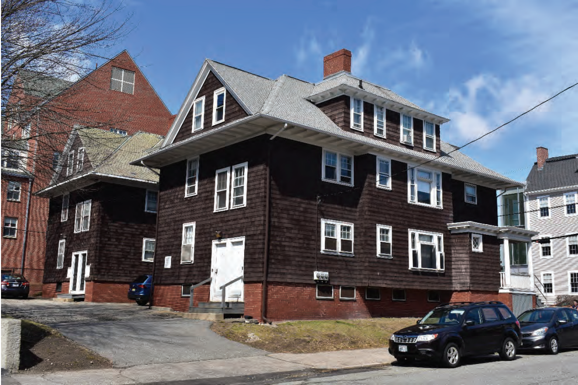
South and east elevations, looking northwest.
